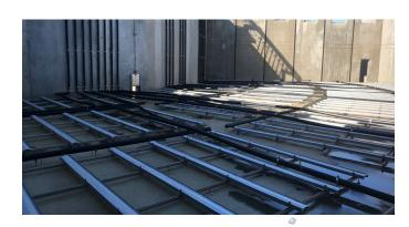
In total, 1,712 AEROSTRIP®s type Q4 are installed in four new aeration tanks.
